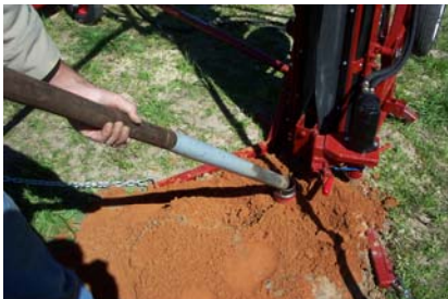
1 Insert split spoon sampler with respective amount of drill rod into hole. The ring at the top of tower may be used to guide/hold drill rod string when inserting into hole.
