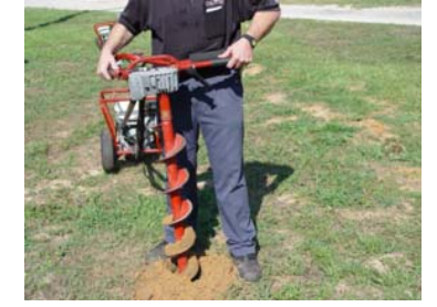
8 When hole is complete stop auger and pull out for clean hole.
