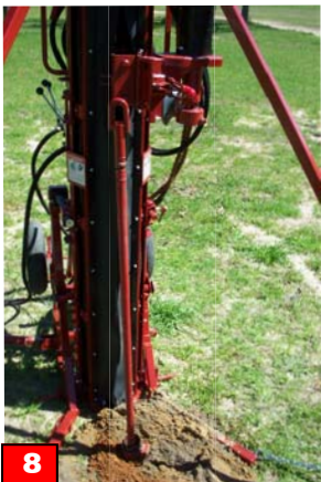
8 Reinsert center rod string with additional center rod and center rod puller attached.
