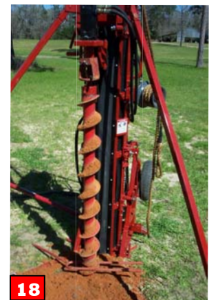
18 Raise auger string until the second (from top) hollow stem section can be held in position with auger fork/stop.
