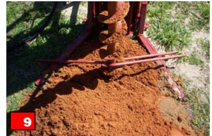
9 Once desired depth is reached, raise drill string to top of stroke. Insert auger fork (stop) around auger (extension) barrel approximately 6-8 inches below the top of the auger (extension).
